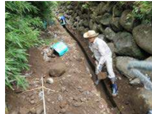
Removal of sediment from waterways in Kurogi, Yame city, Fukuoka in 2012's flood disaster.
