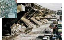
Collapsed viaducts of expressway
