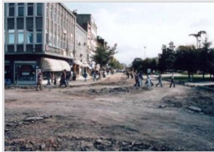
After the earthquake
