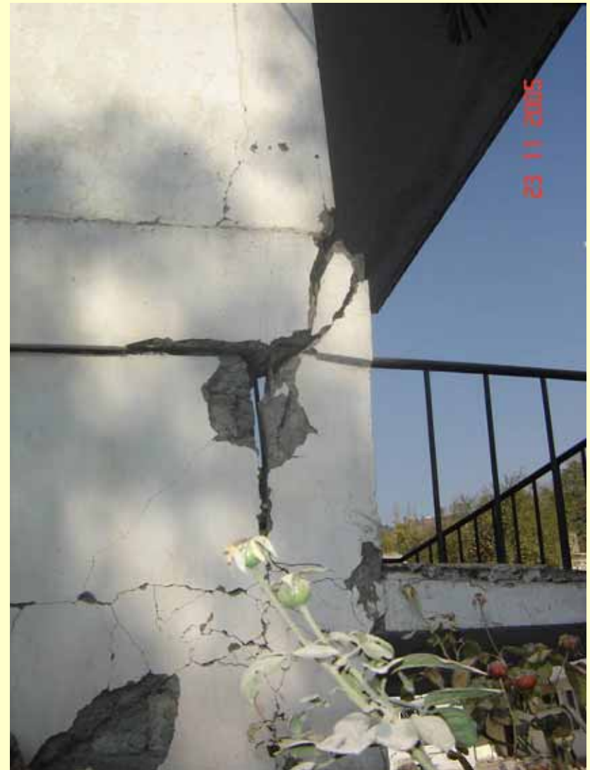
Shear Failure of Joint
